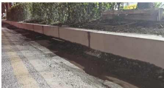
General road drainage system
