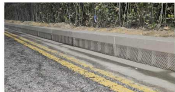
The Drainage & Clean system for green roads
